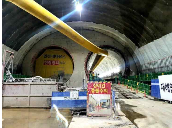
(b) TBM관통 전경
