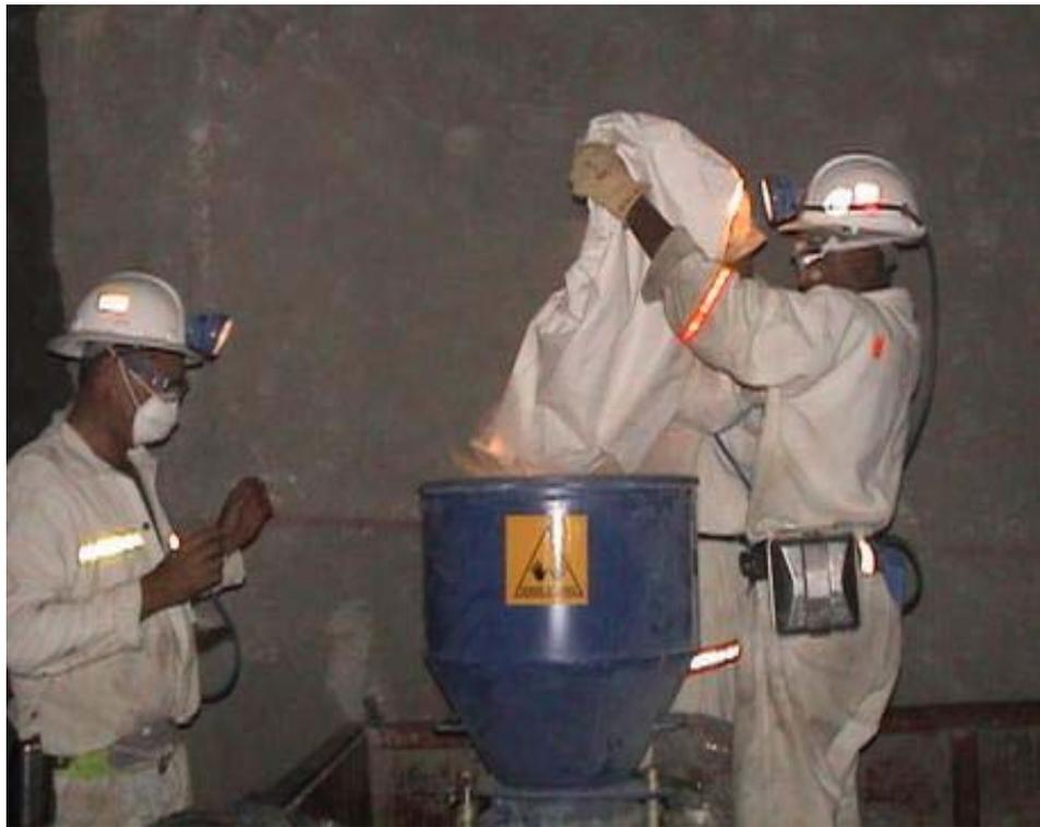
(a) Batching and mixing of TSL
